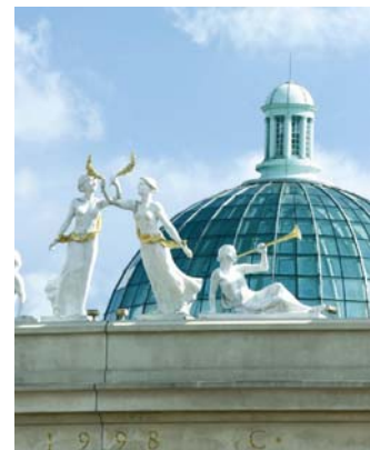
The Trafford Centre, Manchester
